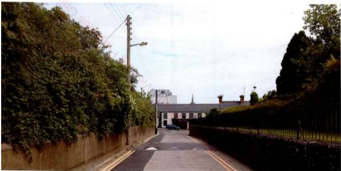
Figure 1: Entrance Walls Looking East towards Georges Street.
